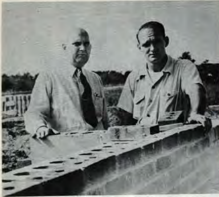
George K. Rosenquist and his son, Kent, of The Village China Shop, pause in their inspection of progress on the roadside china and glass store they are building on West Auburn road.
