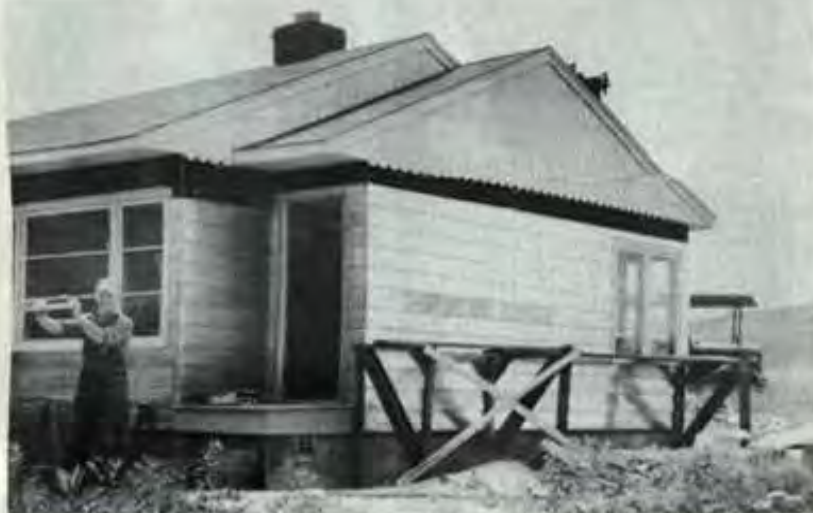
Morse Darling unloads lumber for a new house on East Tienken Road.
